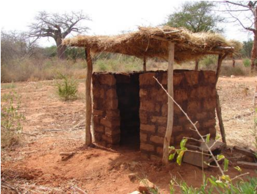
A newly completed latrine in Kenya. Credit: computerwhiz417
