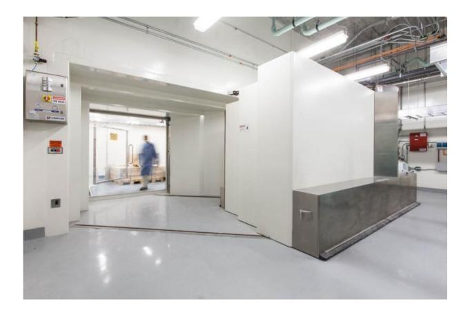
The rail door that leads to the cyclotron, a type of particle accelerator that helps make radioactive materials for a new kind of imagining.
