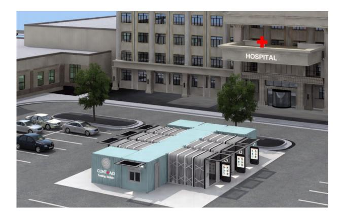
The design of the facility is made up of 10-foot shipping containers and prefabricated expandable units. The setup of the structure is designed to be quite simple with minimal on-site preparation, so hospitals can construct it quickly and efficiently, or even move it if the need arises. Credit: Florida International
