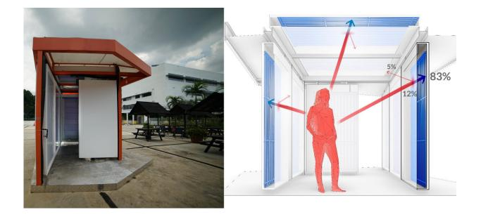
The "Cold Tube" pavilion (left) during tests in Singapore in January 2019. The structure is able to provide a cool and comfortable outdoor space through the use of radiant cooling (right). Credit: photograph: Lea Ruefenacht; diagram: Dorit Aviv and Jiewei Li
