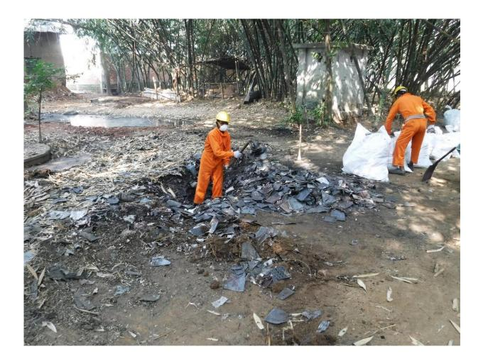
Workers dig up contaminated soil and waste at the site of a former lead battery recycling operation in Kathgora, Bangladesh. Credit: Pure Earth
