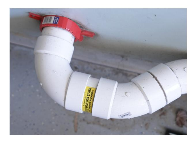
Experts say the only way to know if there are high levels of radon in your home is to test for it. Radon is the leading cause of lung cancer among non-smokers, but a remediation system can safeguard your home by diverting this cancercausing gas outside. Credit: The Ohio State University Comprehensive Cancer Center
